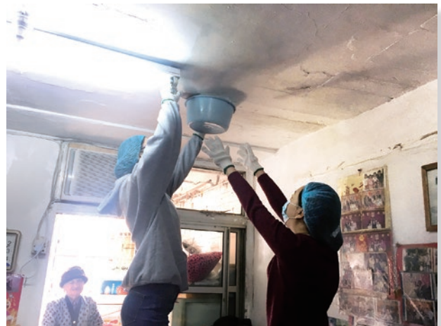
Refurbishing homes of the elderly. 為長者粉飾家居。
