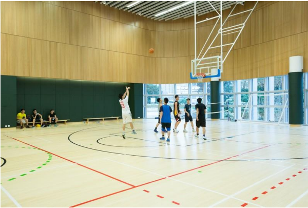
Bamboo Floors in the Sports Hall
